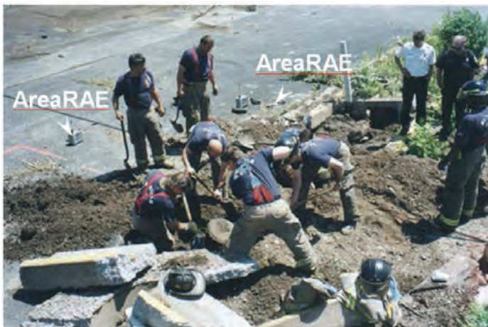
Figure 3. Perimeter monitoring during repair of leaking gas pipe (propane is explosive, but not highly toxic).
